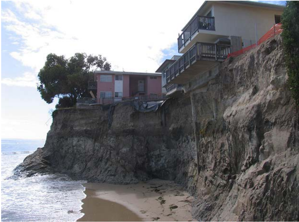
Eroding bluffs in Santa Barbara
