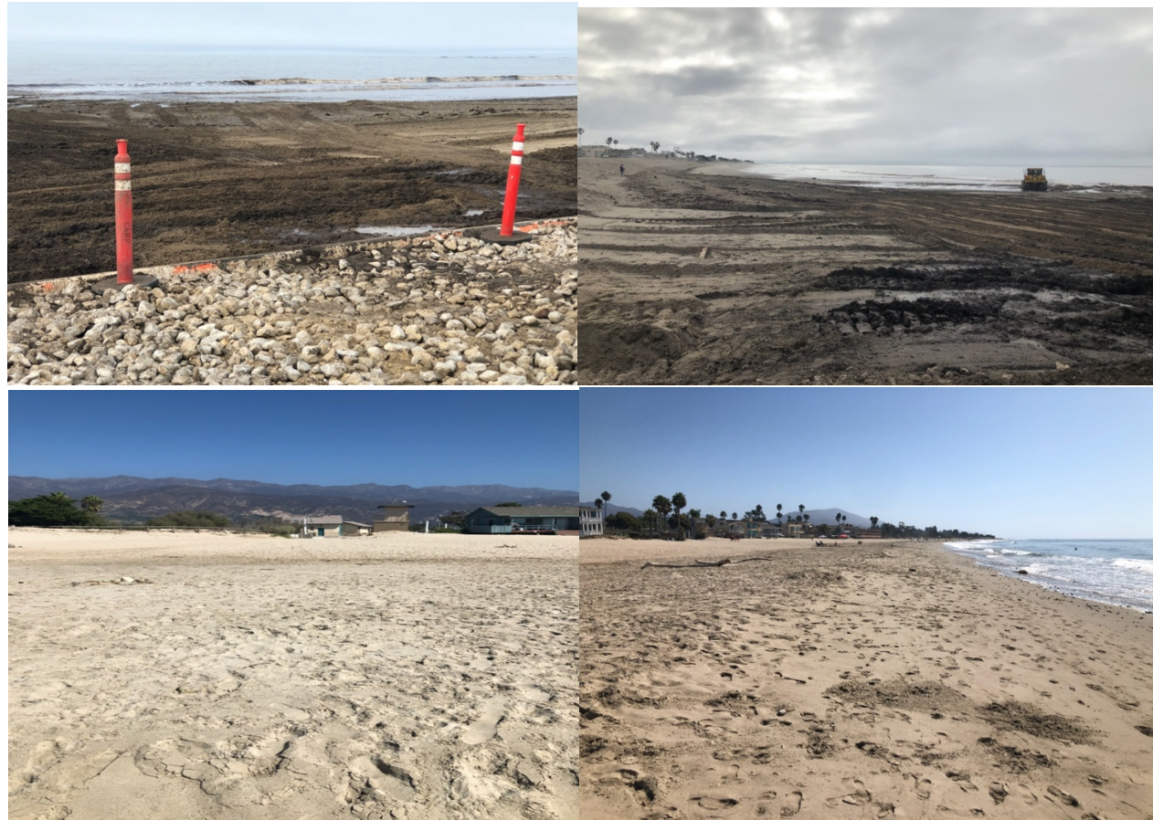
Carpinteria City Beach During Beach Nourishment and After Beach Nourishment: 2019
