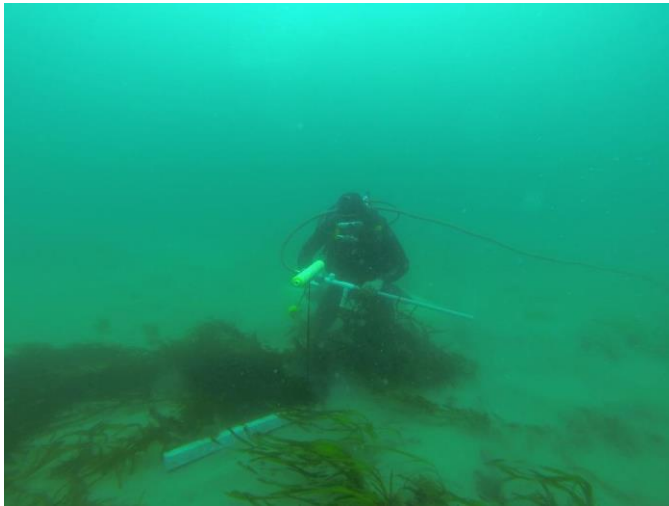
Column with descender sitting on seafloor. Bob Kiel getting ready to water jet hole into seafloor for column.
