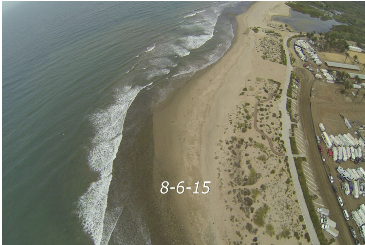
Surfers Point Phase 1 Cobble, sand beach and dunes 'Living Shoreline' and new bike path moved out of hazard zone
